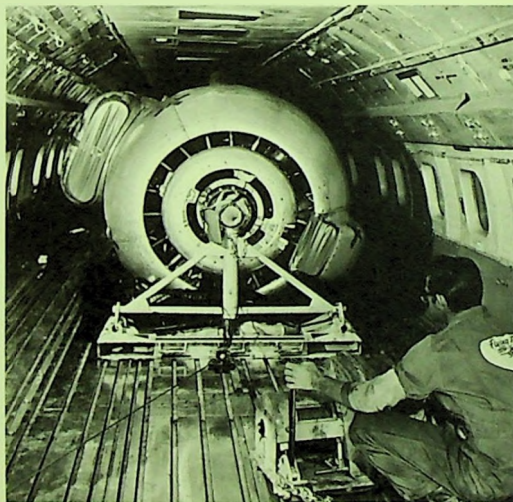
With this electrically-powered winch, secured to the aircraft floor, a huge airplane engine is quickly and smoothly pulled into tie-down position aboard a Tiger airfreighter. Such equipment greatly expedites loading of heavy freight, a specialty of Tiger service.
