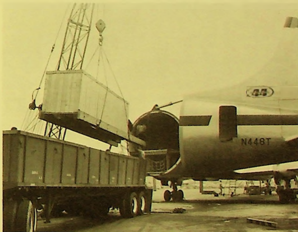
Burbank, Calif.—Generator is unloaded into flat-bed truck.
