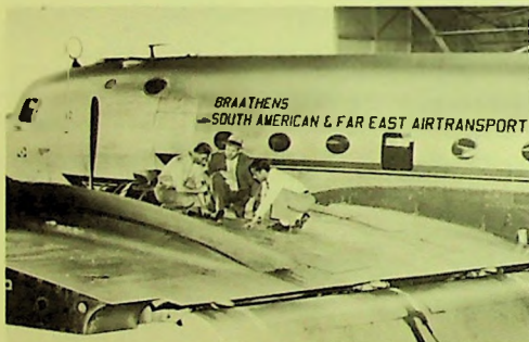
Engineering, modification and overhau
