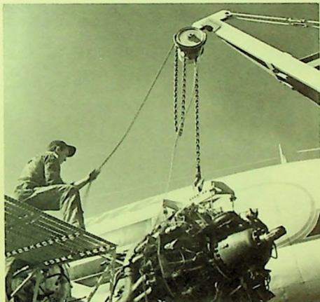
A routine engine change on a C-46.
