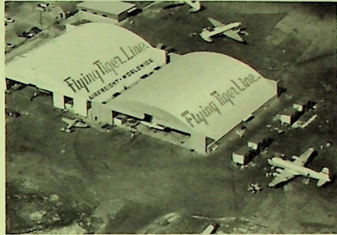
Aerial view of the expanded maintenance and cargo handling facilities at Burbank, California.
