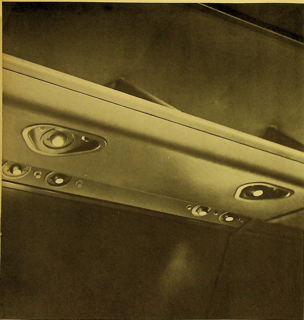
A detailed view of the removable hat rack equipped with individual passenger reading lights and stewardess call buttons.
